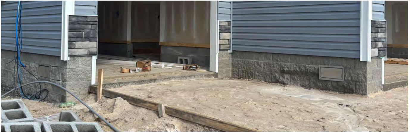
ENGINEERED FLOOD VENTS IN SIDE OF GARAGE.
