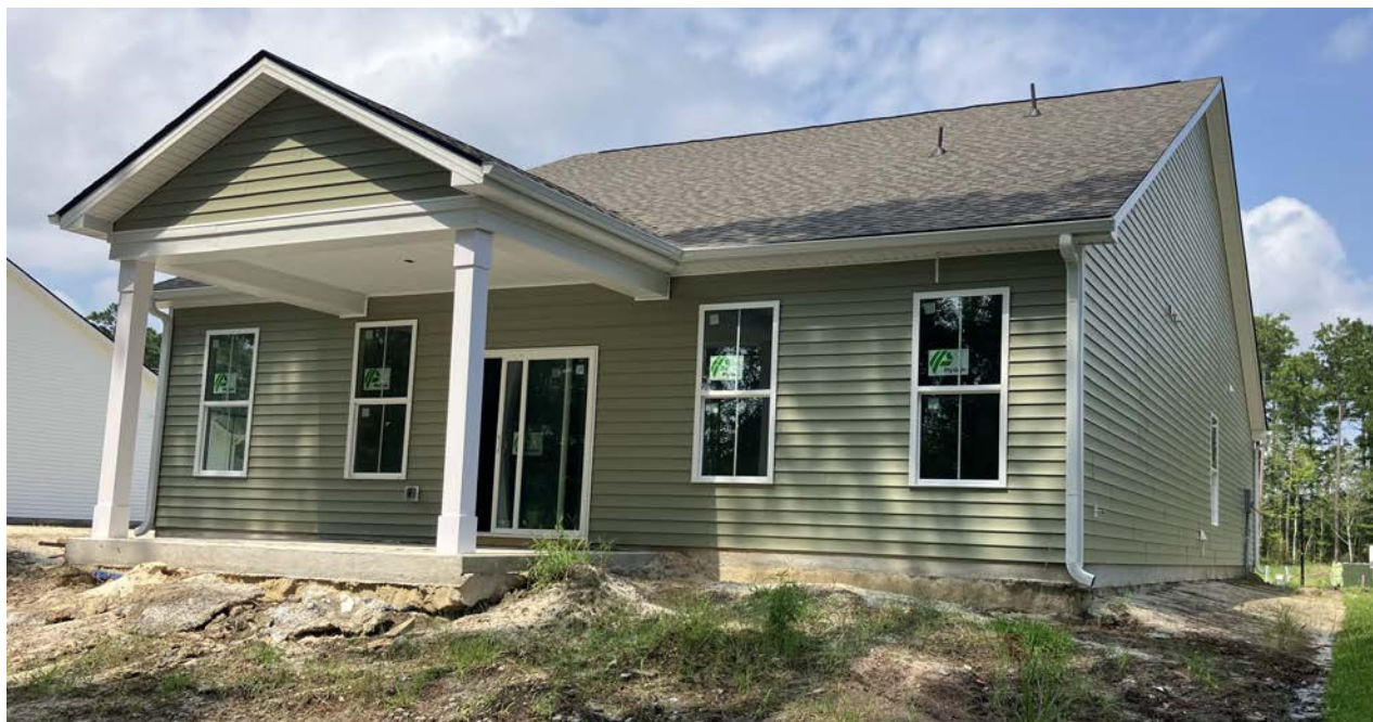
Photo Four Caption: REAR LEFT VIEW 08/12/2024
