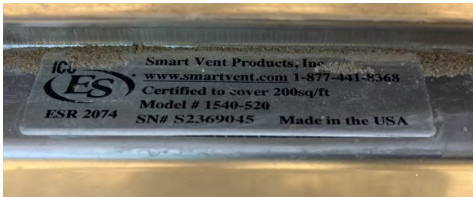
FLOOD VENT IN SIDE OF GARAGE MODEL NUMBER
