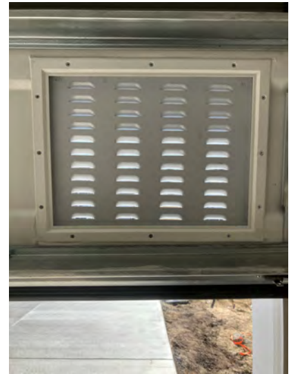
BACK OF NON-ENGINEERED FLOOD VENT
