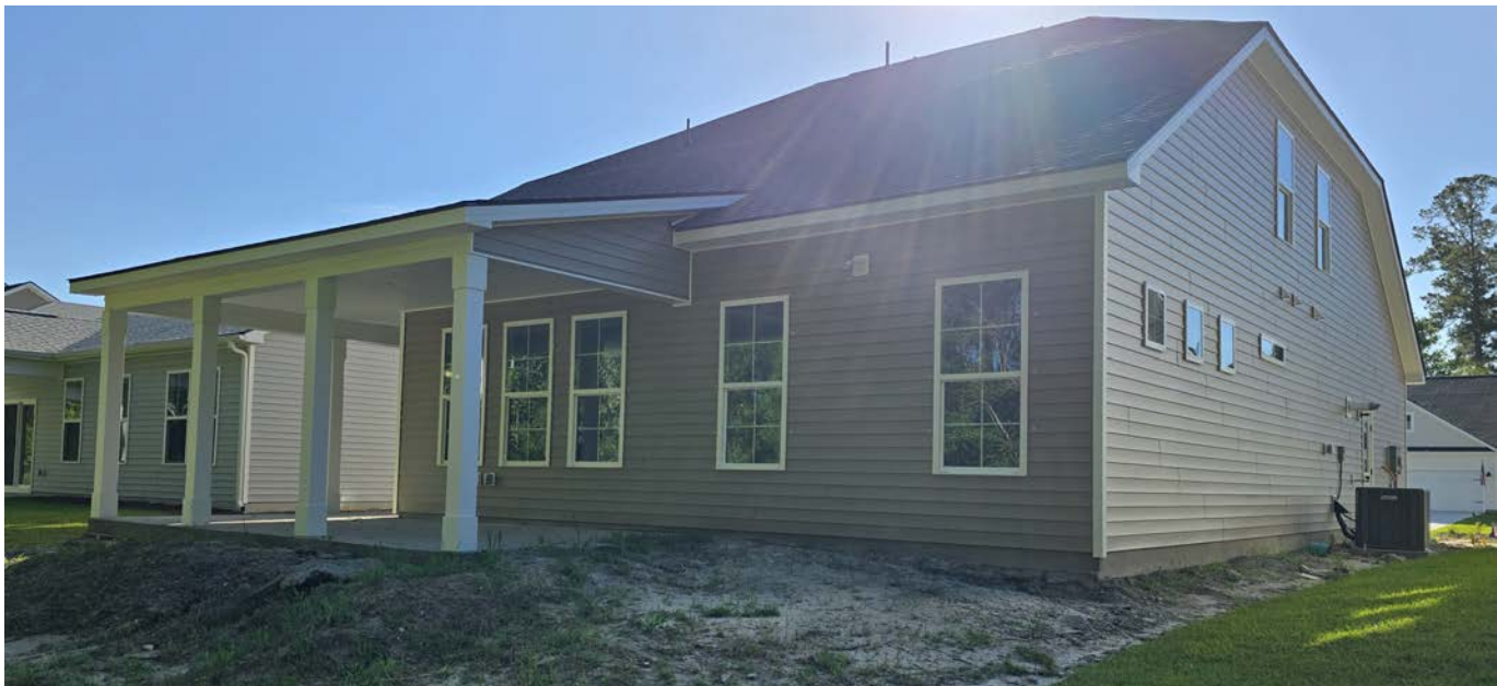
Photo Four Caption: REAR LEFT VIEW 05/14/2025
