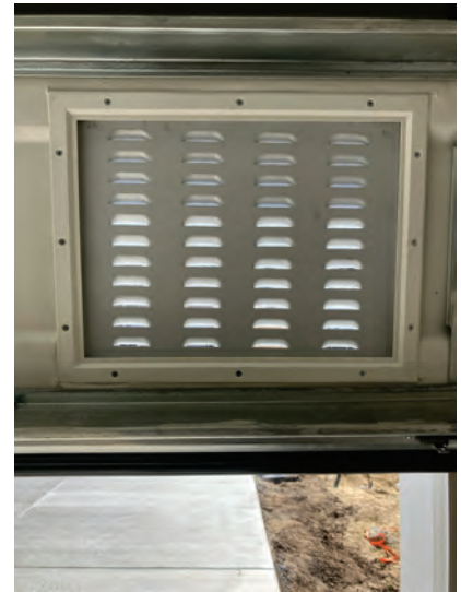
BACK OF NON-ENGINEERED FLOOD VENT
