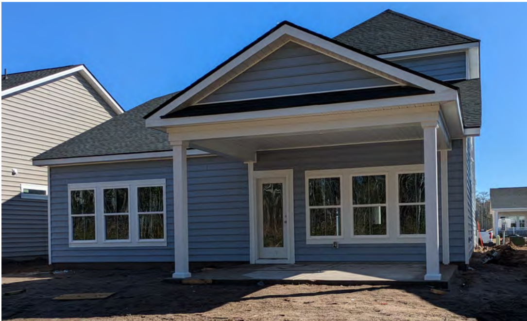
Photo Four Caption: REAR LEFT VIEW 01/28/2025
