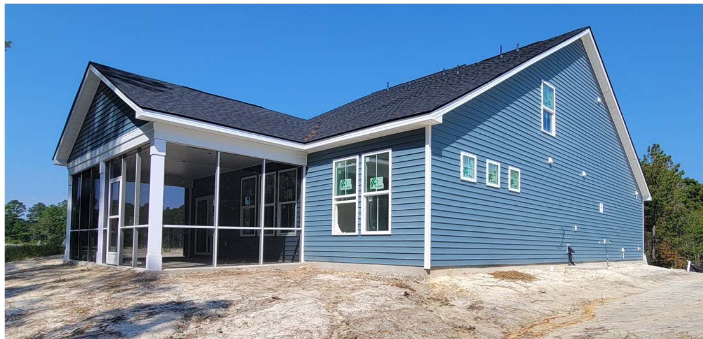
Photo Four Caption: REAR LEFT VIEW 10/08/2024
