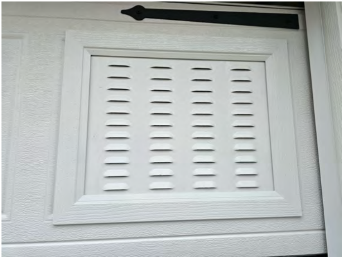
NON-ENGINEERED FLOOD VENT IN GARAGE DOOR - FRONT
