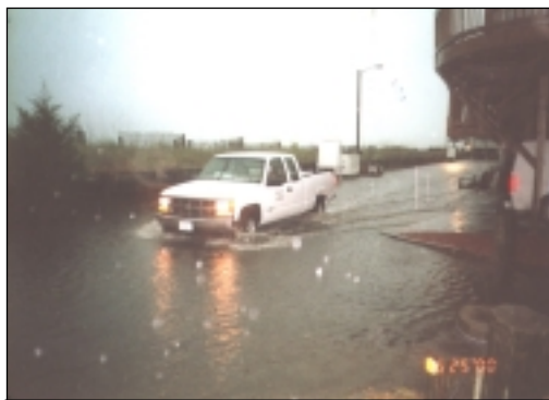
Flooding Near HC SBD01-00 during Rain Event
