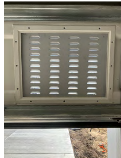
BACK OF NON-ENGINEERED FLOOD VENT
