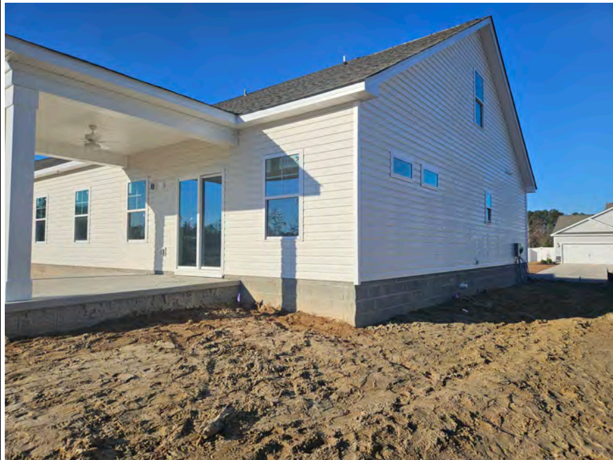
Photo Four Caption: REAR LEFT VIEW 12/01/2023
