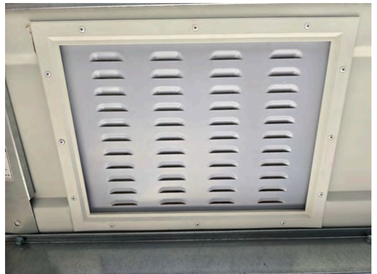
BACK OF NON-ENGINEERED FLOOD VENT IN GARAGE DOOR
