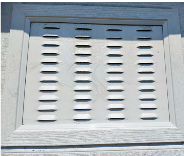
FRONT OF NON-ENGINEERED FLOOD VENT IN GARAGE DOOR
