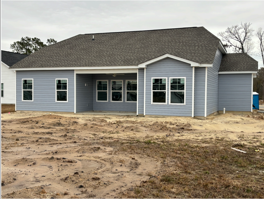
Photo Three Caption: REAR VIEW 01/14/2024
