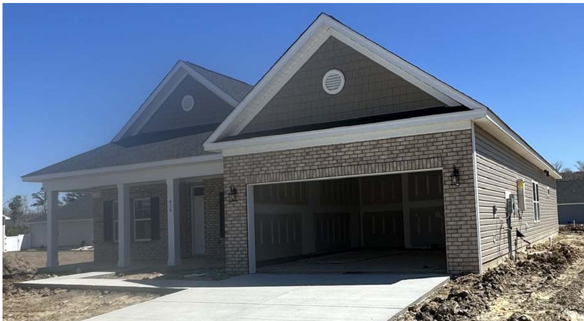
Photo Two Caption: FRONT LEFT VIEW 03/25/2025
