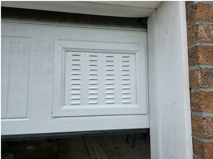
NON-ENGINEERED FLOOD VENT IN GARAGE DOOR (FRONT)
