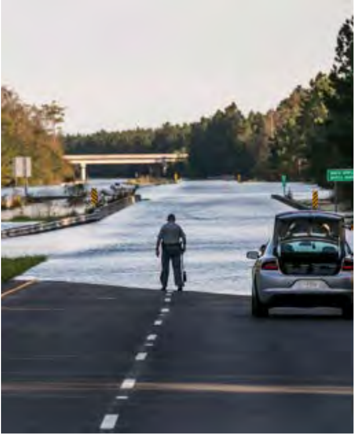
Flooding in Conway following Hurricane Florence in 2018 Source: ABC 4, 2018.
