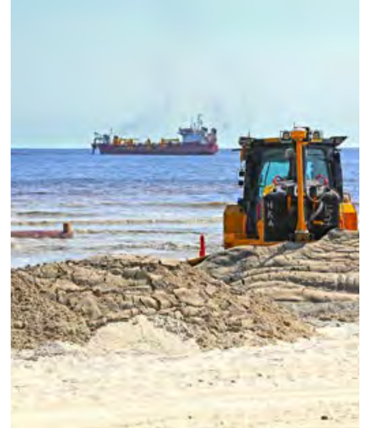
Myrtle Beach Renourishment Project after Hurricane Florence Source: USACE, 2018.
