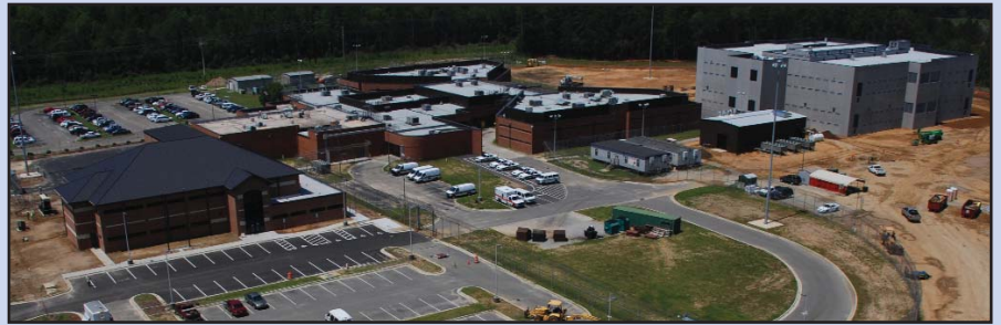
NEW J. Reuben Long Administration BUILDING (L) AND RANDY GERALD TOWER
