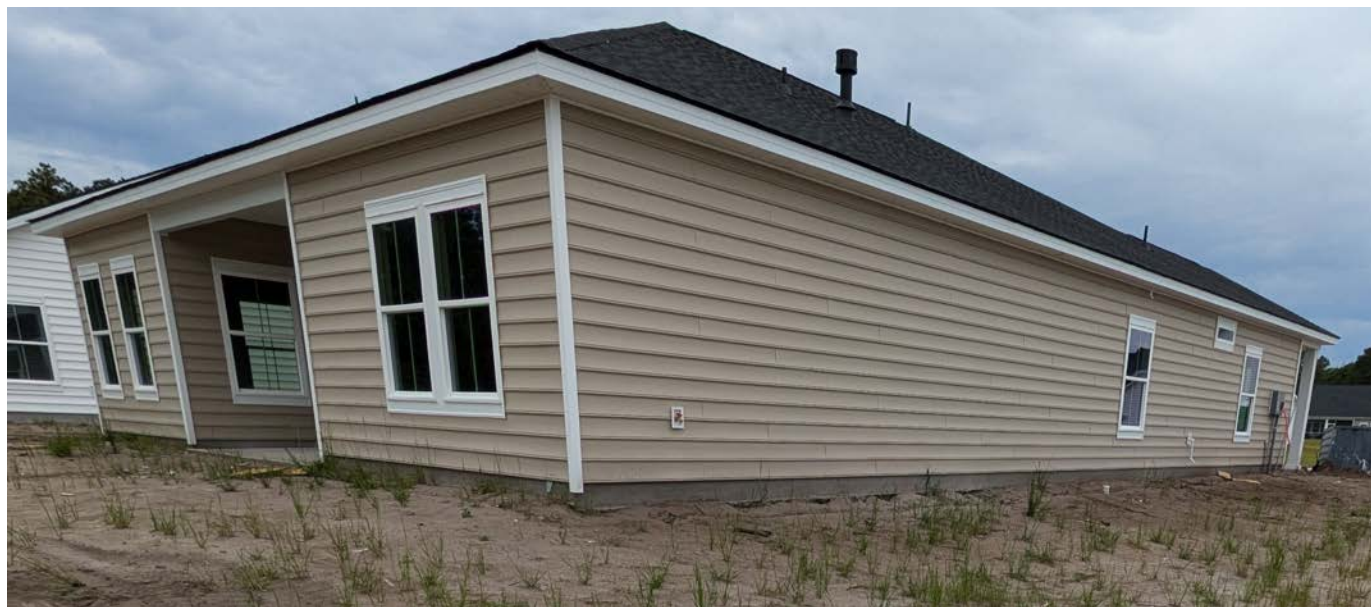
Photo Four Caption: REAR LEFT VIEW 05/07/2025
