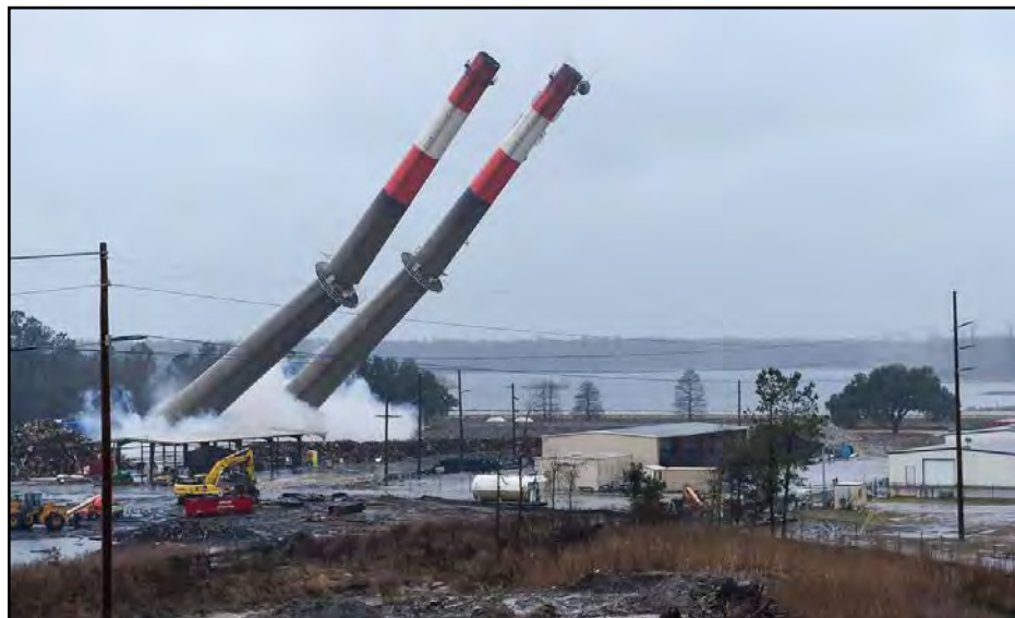
Demolition of the Granger Generating Station stacks Photo Credit: Jim Huff, Santee Cooper
