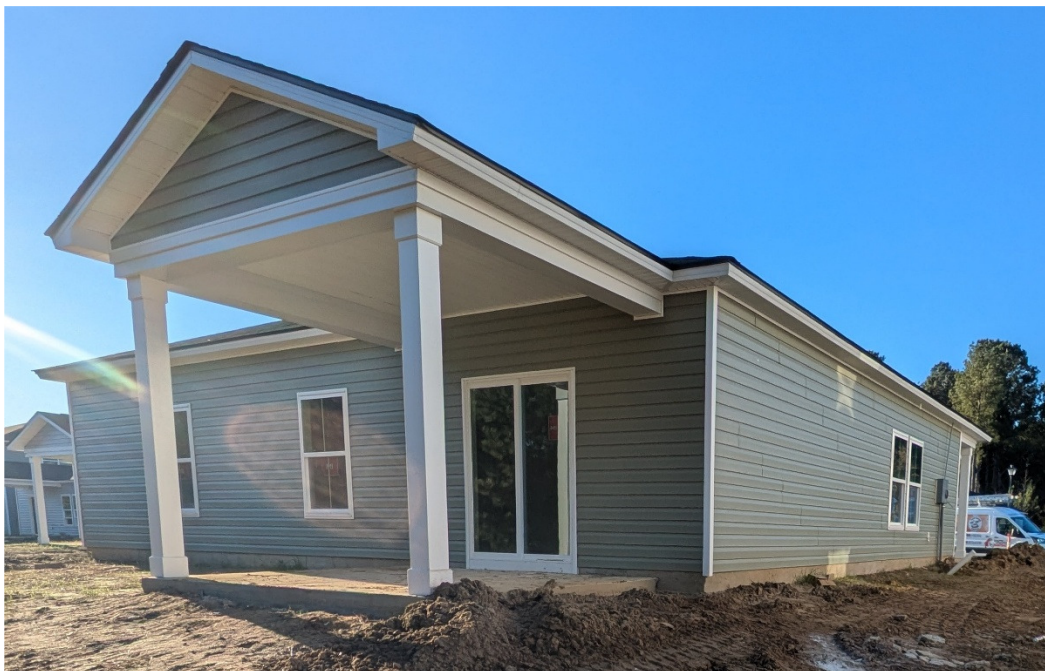
Photo Four Caption: REAR LEFT VIEW 12/18/2025
