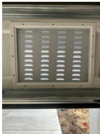
BACK OF NON-ENGINEERED FLOOD VENT
