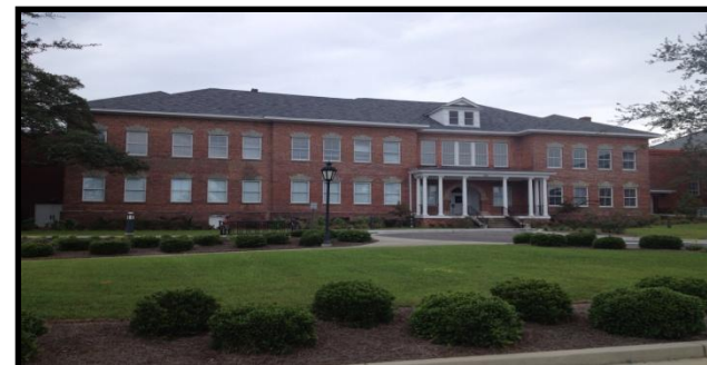
Burroughs School Building 2012
