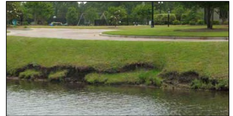
Pond Bank Erosion
