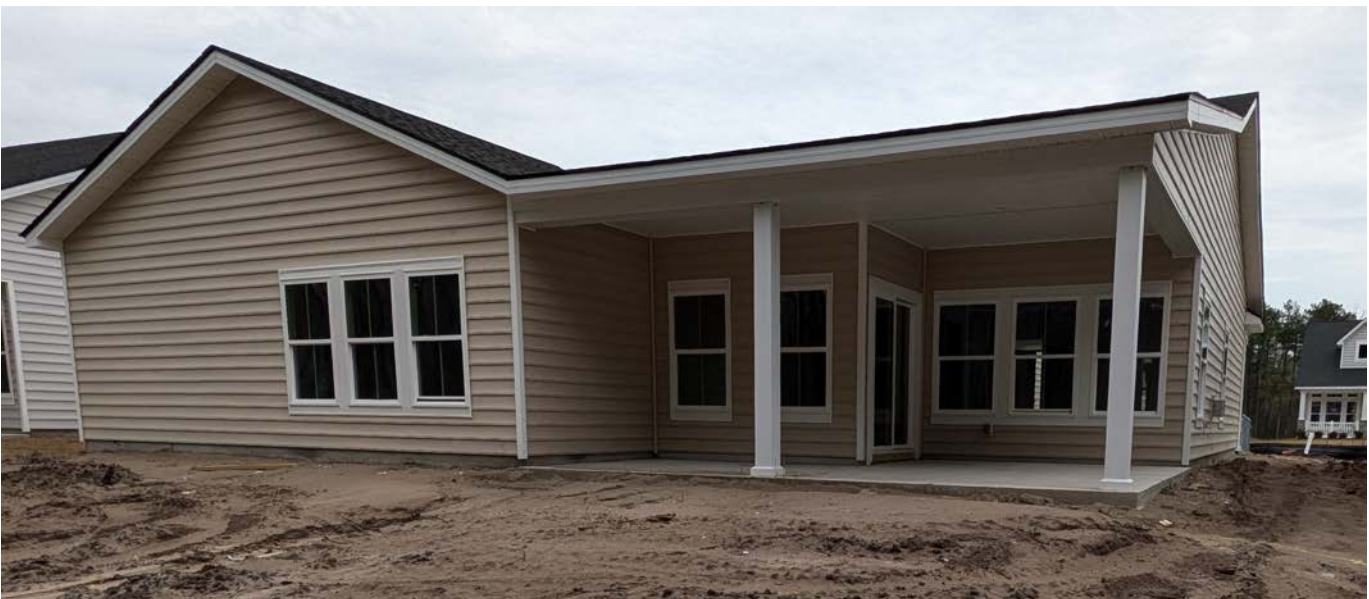
Photo Four Caption: REAR LEFT VIEW 03/24/2025
