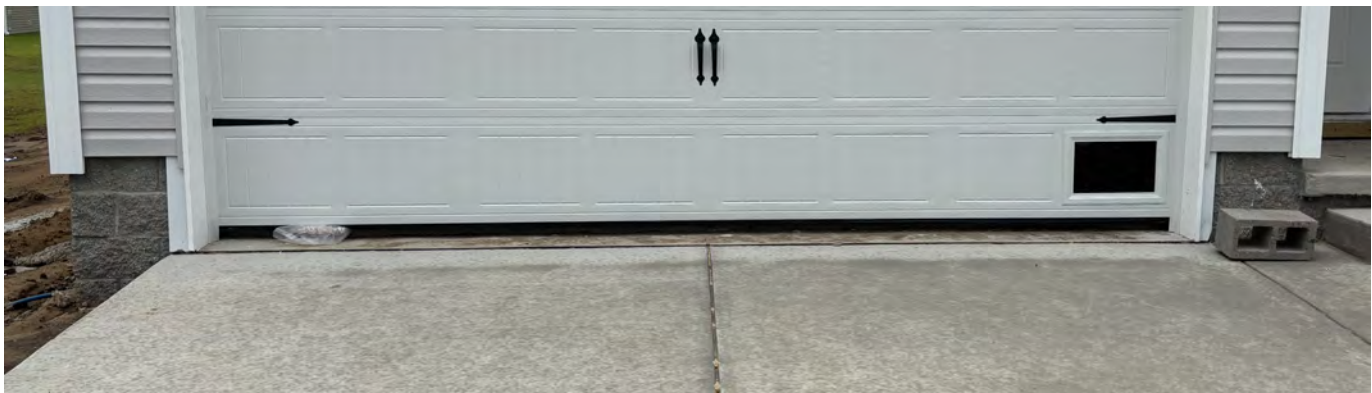
1.4'x0.9' OPENING IN GARAGE DOOR
