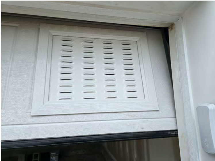
NON-ENGINEERED FLOOD VENT IN GARAGE DOOR (FRONT)
