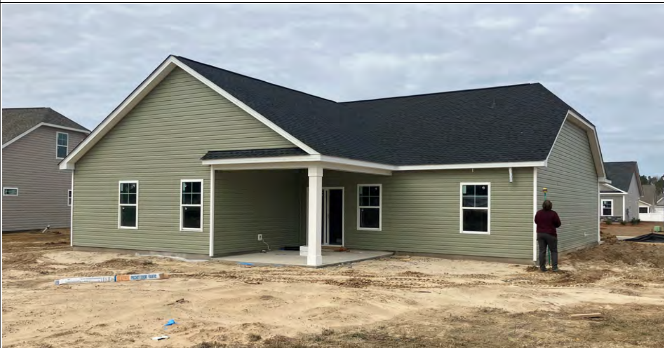
Photo Four Caption: REAR LEFT VIEW 01/24/2024
